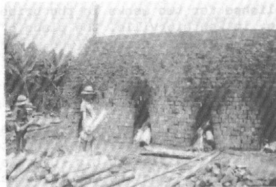
Brick making (burning in kiln)
