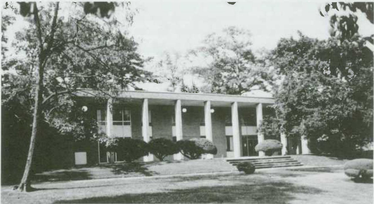
The Fine Arts Building at Oakwood College
