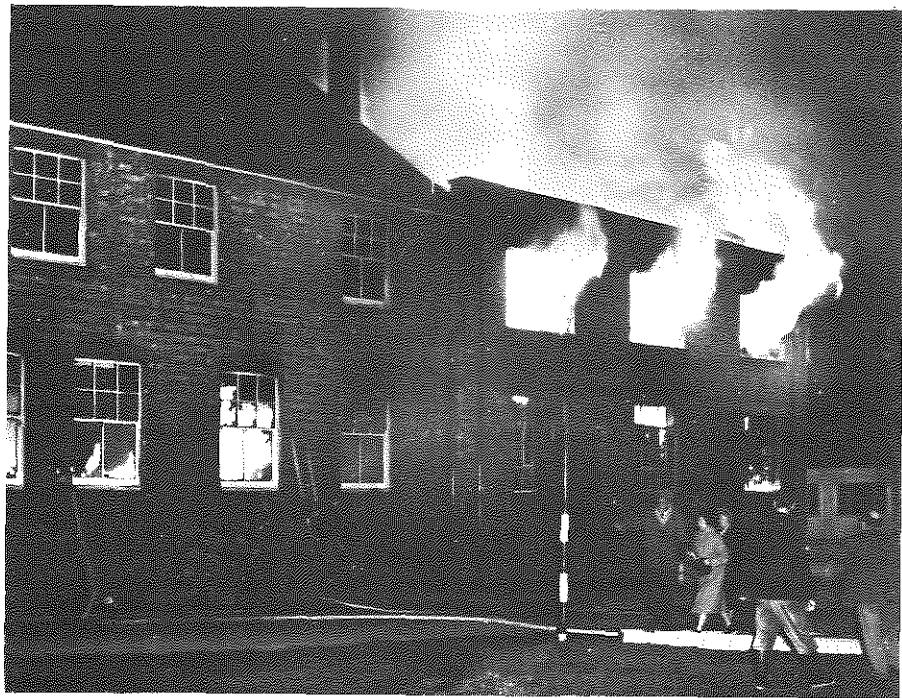
The Stanborough Press fire of January 3, 1964, which destroyed much of the administrative block.
