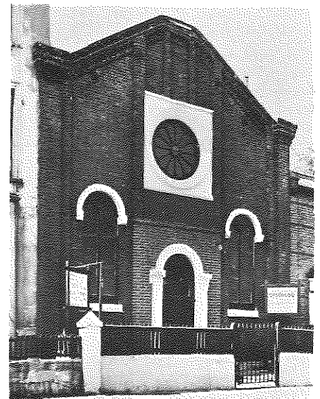
Duncombe Hall Training College (1902-4) London, where ministerial training began in Britain. It is now a church.
