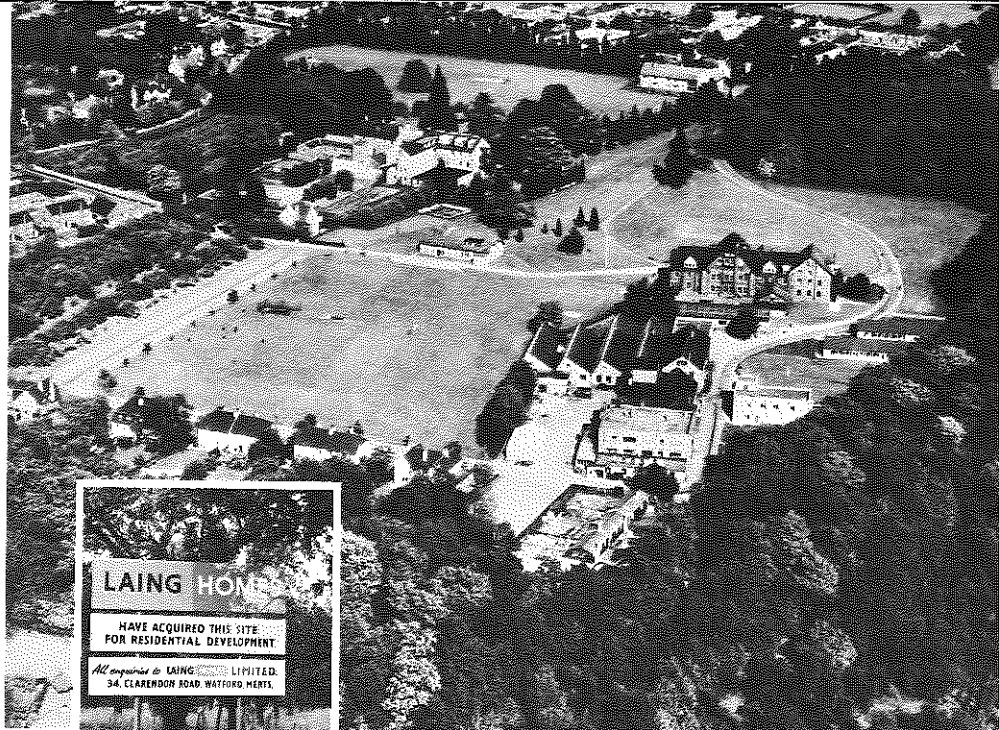
Aerial view of Stanborough Park, Watford, 1962. Inset: Part of Stanborough Park orchard sold for development D (see map below).
