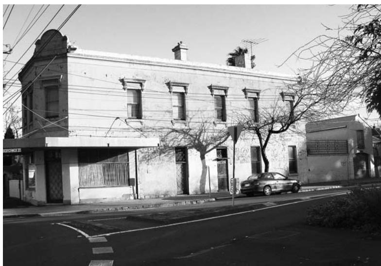
Burnham House, former Mission Home and Printing Office for Bible Echo & Signs of the Times, Cnr of Scotchmer and Rae Streets, North Fitzroy.
